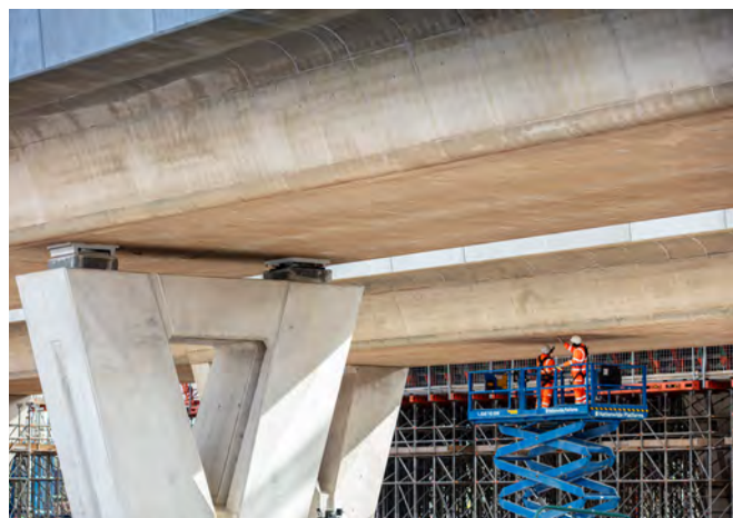
Working under the deck of HS2's Curzon No 3 viaduct in Birmingham.
