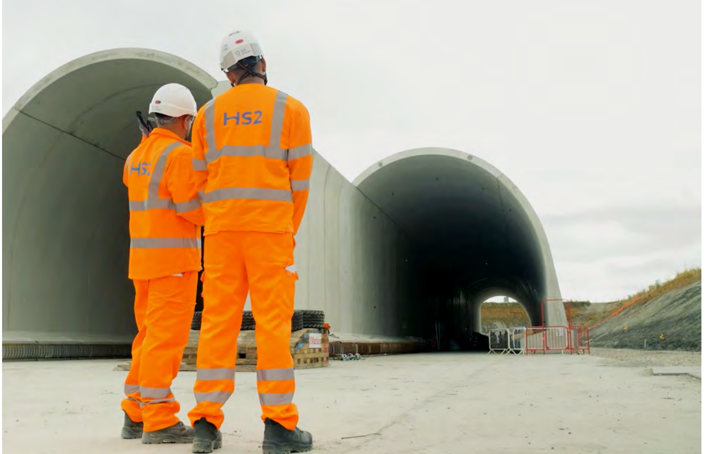
First completed sections of the Chipping Warden 'green' tunnel.
