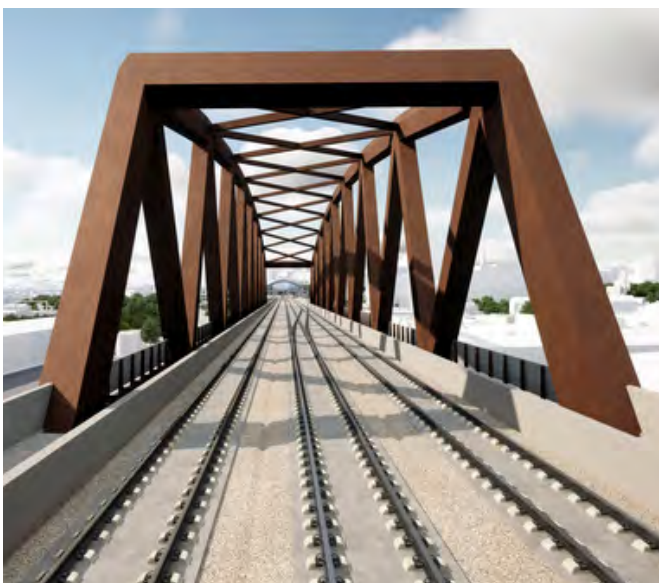
Track view of Curzon No 2 viaduct in Birmingham
