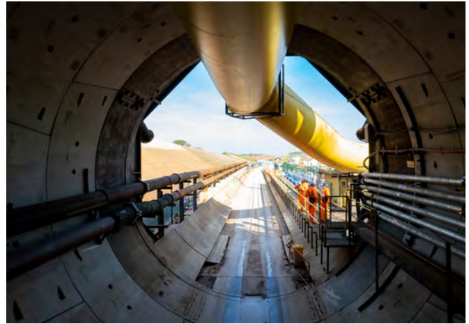
Inside HS2's tunnel at Long Itchington Wood in Warwickshire
